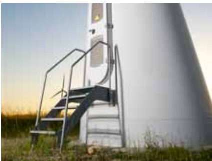
Wind tower installation application
